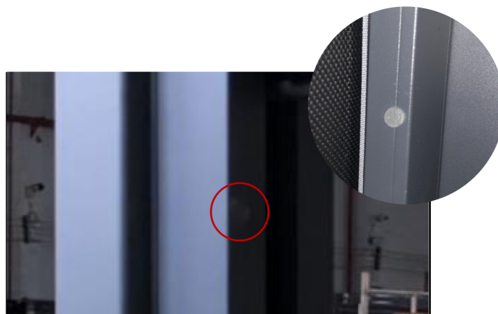
12. After the track fixing screws are tightened, plug the screw holes with rubber plugs
