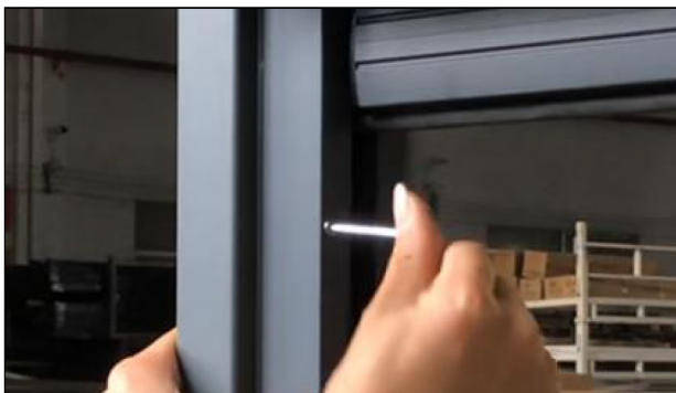
11. After assembling the complete track, lock the track with the hex wrench
